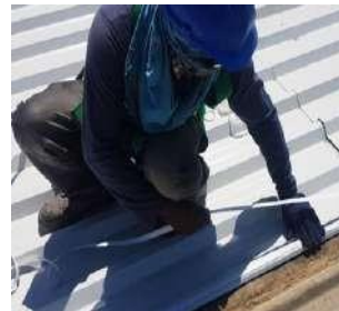
METAL DECK ROOFING SYSTEM
