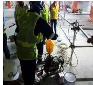
CONCRETE REPAIR & INJECTION SYSTEM
